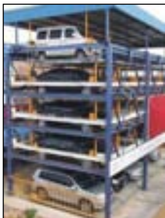
Typical Layout of Multi-level Puzzle Car parking
