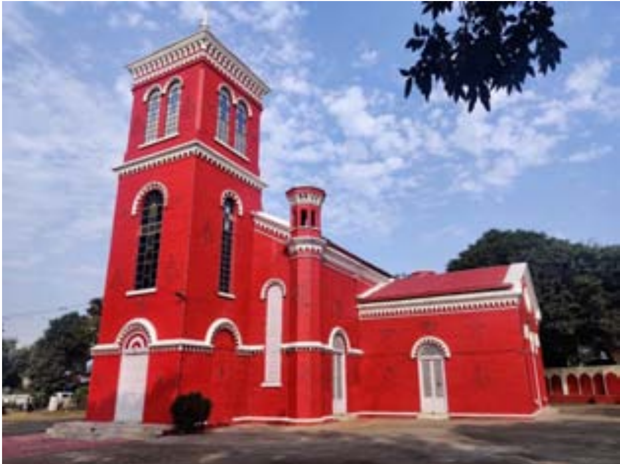
Figure 37 Christ Methodist Church – Civil Lines, Bareilly
