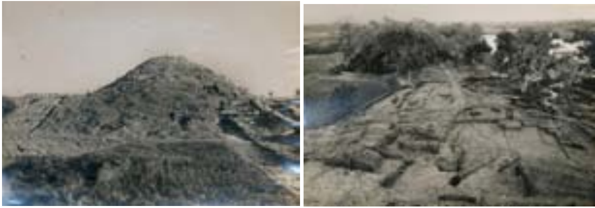
Figure 22 Archival image of the site excavation activities (1940 – 1945) Alexander Cunningham
